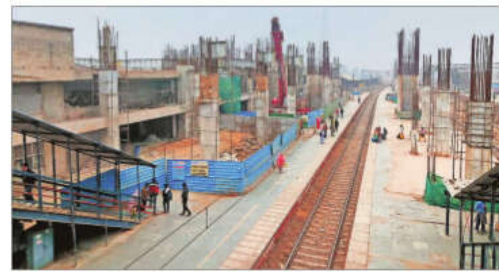
Faridabad station redevelopment work almost 50% complete. DHEERAJ MISHRA
